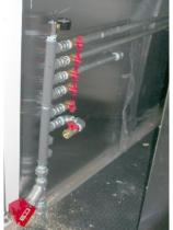
repairs by closing the shutoff at the manifold. Appliances often have pilot lights. Make sure the manifold valve that corresponds with that appliance is on the "off" position until you are ready to light the appliance. When you are ready, open the manifold valve and immediately light the appliance. DO NOT LEAVE MANIFOLD VALVES OPEN UNLESS YOU ARE USING THAT APPLIANCE!
