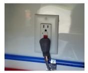
breaker will trip. You simply need to press the reset button on the outlet to reset it. You need to push the button in with a screwdriver or pencil to get it to reset.
