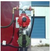
**Regulator** - Your regulator reduces the pressure from the tanks to a correct pressure for your equipment. If there are shutoffs in the line between the tank and the regulator, they will have to be opened for the tank side you wish to use, to let the regulator get gas. There is typically a shutoff after the regulator which will keep any gas from going into the truck or trailer. This shutoff must be opened for gas to reach your equipment.
